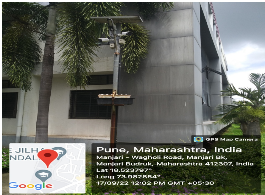
CCTV camera at A Building
